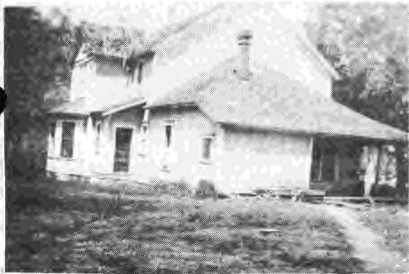
Henry Thiessen's home (Backdoor view)
