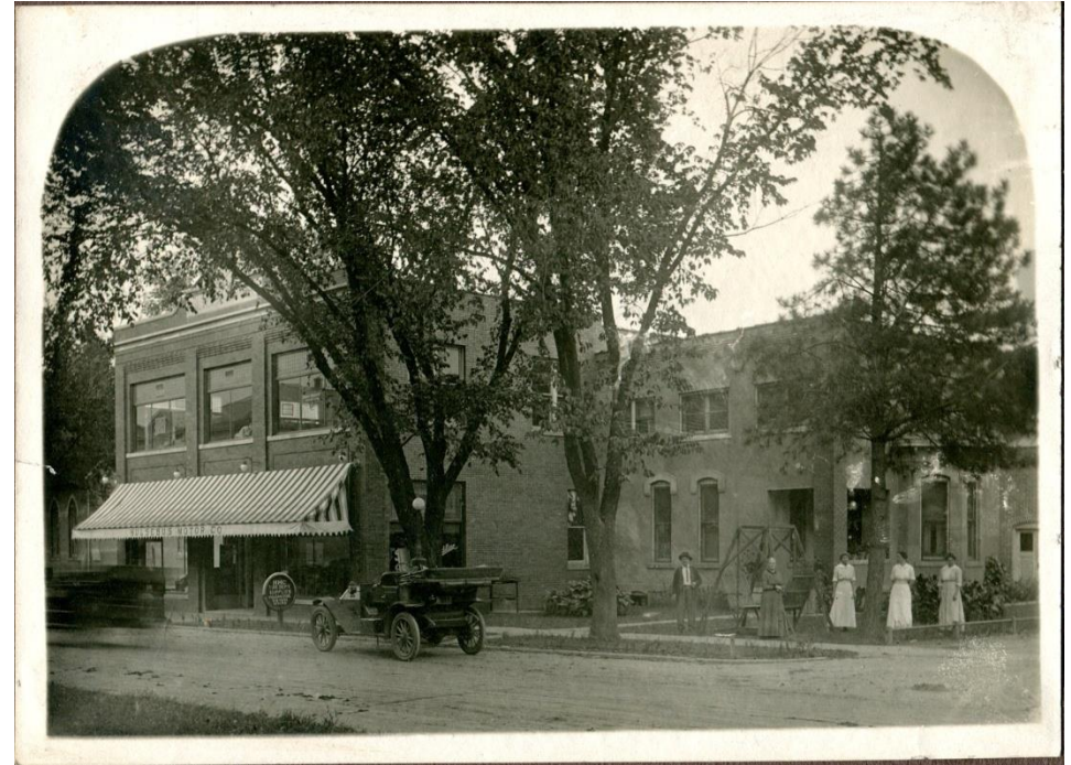
Hulsebus Motor Company, corner of 7 th and Durant Streets
