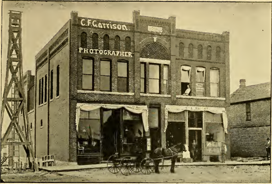
BRICK BLOCK OF C. F. GARRISON, PHOTOGRAPHER, AND S. A. BRIGHT, GROCER, ROLFE.
