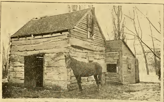
JOHN FRASER'S LOG HOUSE 1868
