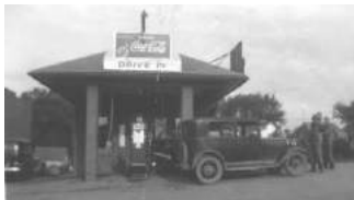
The old Phillips 88 service station in Massena, Iowa, is shown above.
