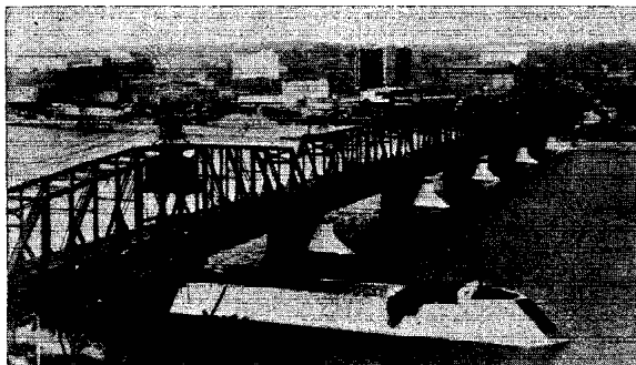
¶This picture of the Rock Island to Davenport bridge is furnished through the courtesy of the Rock Island Railroad. It is a Baltimore truss type, with a swing span. The more modern bridges have lift spans, but this structure, the third on the site, where the first bridge over the Mississippi River was built, still serves the Rock Island Railroad and passenger traffic.
